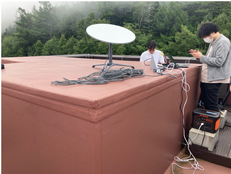
Measurement Gears on Rooftop
