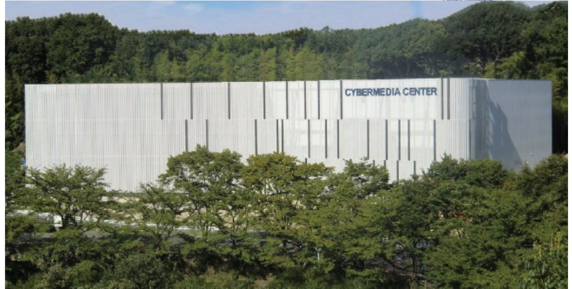
IT core as data center
