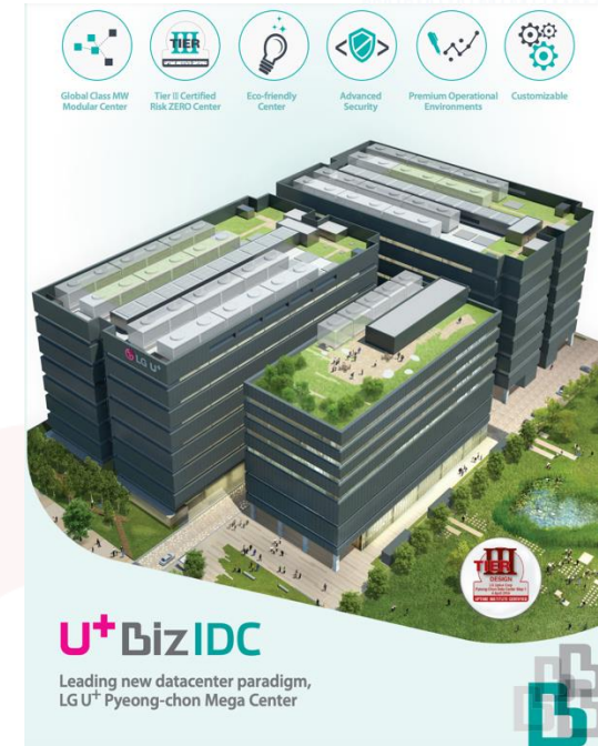
Carrier-neutral Mega Datacenter
